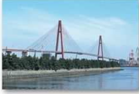
Long-span bridge (Aichi - pref)
